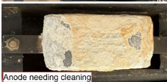
Anode needing cleaning
